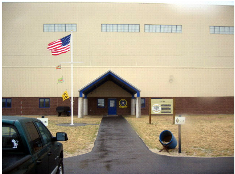
Entrance on North Elevation
