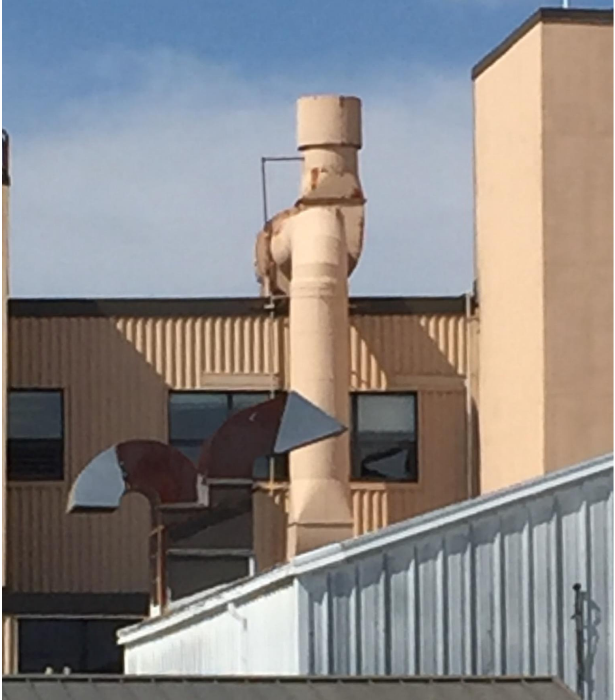
Exhaust off the deck of the roof.
