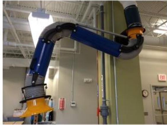
PORTABLE DUST COLLECTION PICK UP ARMS CAN BE MODIFIED FOR ELEVATED TEMP OPS LOCATE ON SUPPLY PLENUMS TO DIRECT ONTO HULL INTERIOR SPACES
