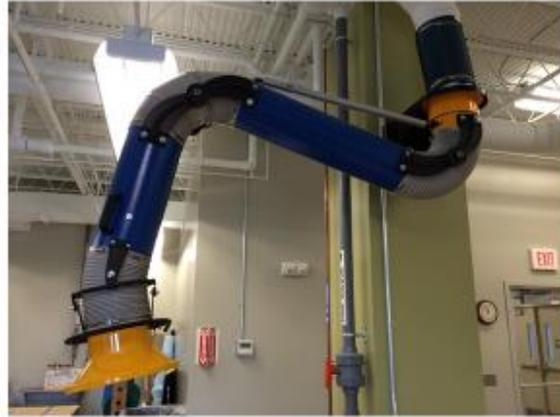
PORTABLE DUST COLLECTION PICK UP ARMS CAN BE MODIFIED FOR ELEVATED TEMP OPS
